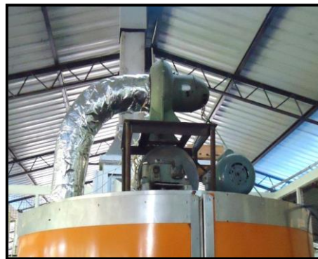
Figure 10: The blower unit has been mounted on top of the bakery oven chamber
